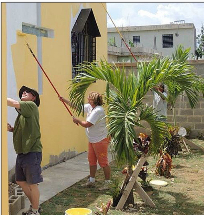
Painting the exterior of the building.
