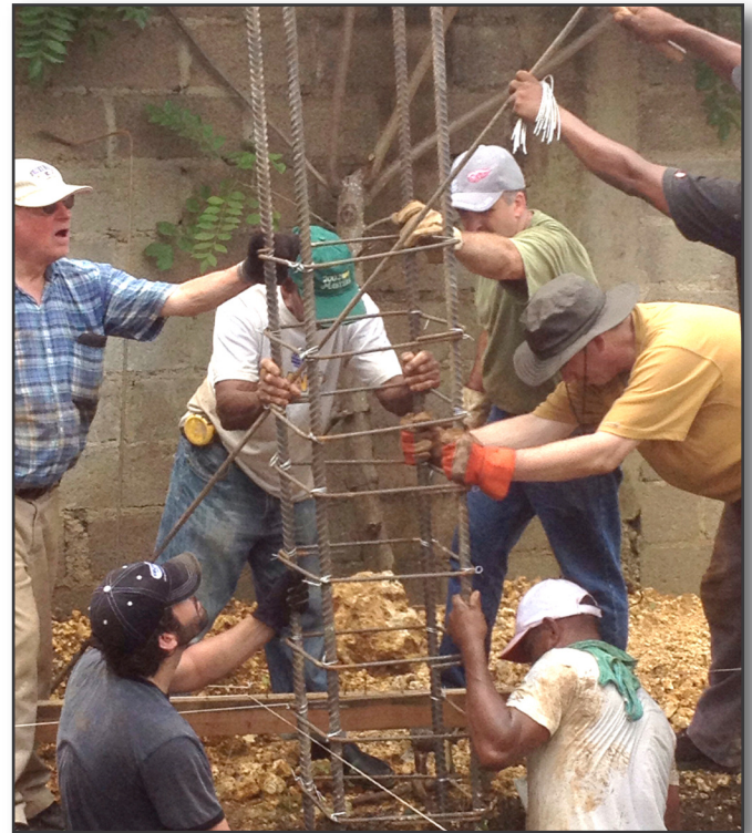
Erecting rebar for pillars.
