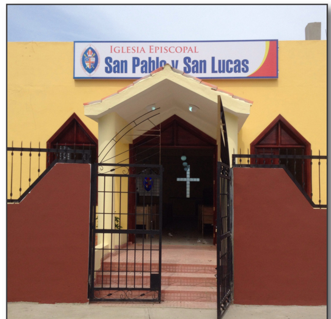
The front entrance of the completed building.
