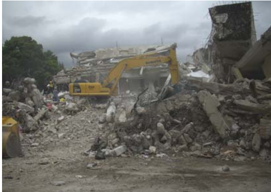
Rubble Removal at Holy Trinity School Complex
